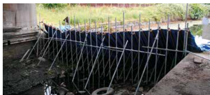
The temporary dam
